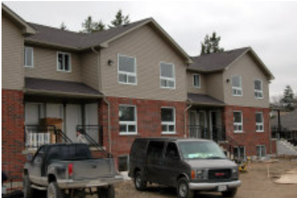
15 new apartments are nearing completion
